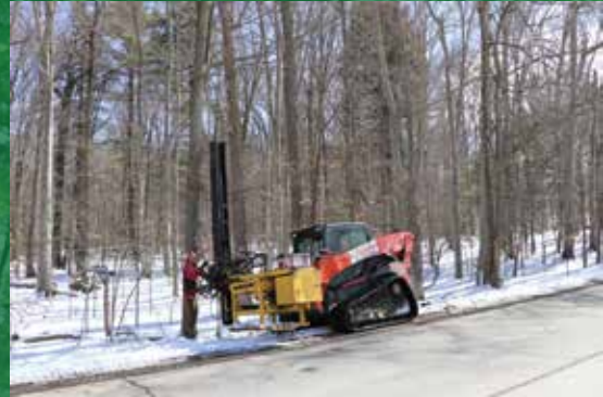
Contractors installing deer fencing along the border of Smith Woods.
