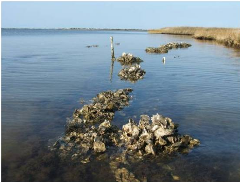
Figure 9.2 Climate change is bringing more extreme storms and damage to coastal regions. Artificial oyster reefs parallel to the shoreline provide a way to slow the rate of coastal erosion by reducing incoming wave energy. They also restore habitat for oysters which have been over-harvested.
