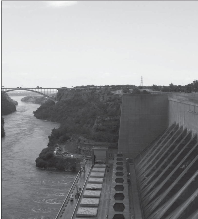
Figure 7.1. Hydropower on the Niagara River. The Niagara River boasts substantial generating power. Ontario's Sir Adam Beck Power Plants (there are two), in this photograph, produce almost 2 gigawatts of electricity and sit across the river from New York State's largest power plant—the 2.4 gigawatt Robert Moses Niagara Hydroelectric Power Station in Lewiston, New York.
