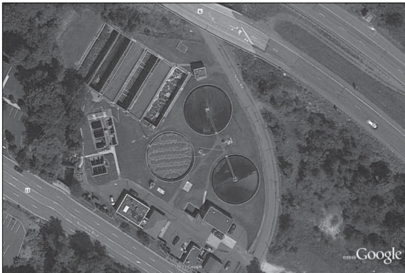
Figure 4.4. The Abington Regional Waste Water Treatment Plant in Chinchilla, Pennsylvania, treats primarily sewage and sewage overflow during periods of heavy precipitation. Like most such plants, it does not accept wastewater from HVHF operations. Treated water drains to Leggetts Creek on its way to the Lackawanna and Susquehanna rivers and eventually to Chesapeake Bay.
