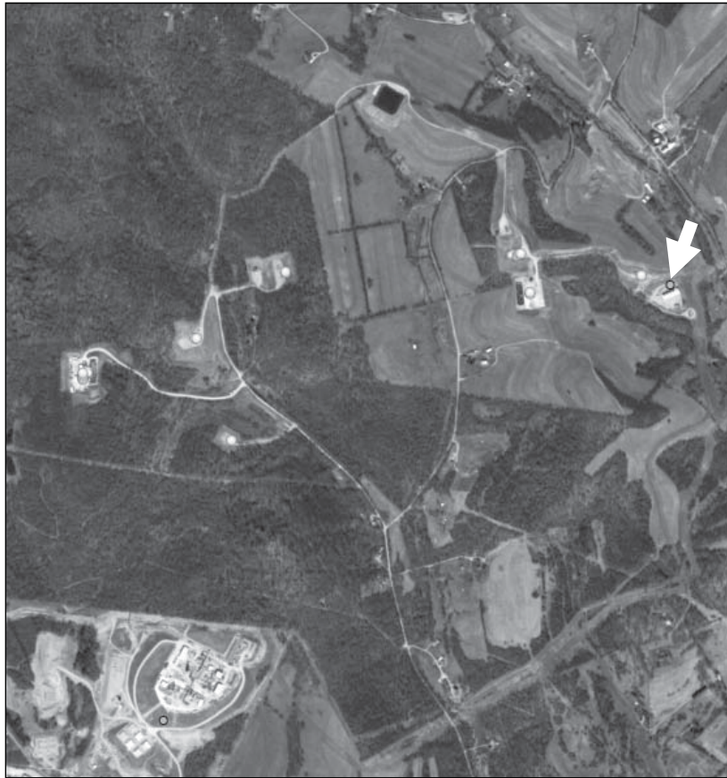
Figure 5.4. Access roads for wells and pipelines lead to habitat fragmentation. This aerial photograph shows HVHF wells and a compressor station in Chartiers Township in Washington County, Pennsylvania. The compressor station (white arrow) sits on a buried pipeline with cleared land above that connects to the nearby wells.
